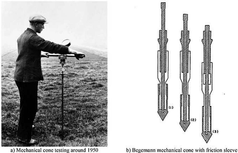
Fig. 1. Early Dutch mechanical penetrometer, from History of Cone Penetration Testing
