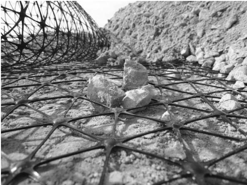
Fig. 1. Hexagonal geogrid for the stabilisation of unbound granular layers
