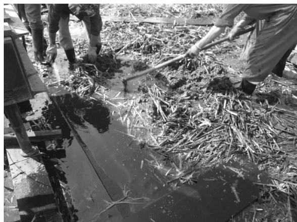
Fig. 7. Careful removal of the roots of the vegetation to provide room for the hammer.
